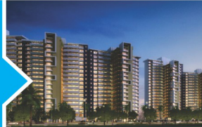
Golf View Apartments (Tulsiani) Lucknow
